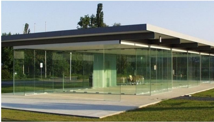
Figure 9: Use of glass as primary structural elements Centre of German Glazing Handcrafters in Rheinbach, Germany.
