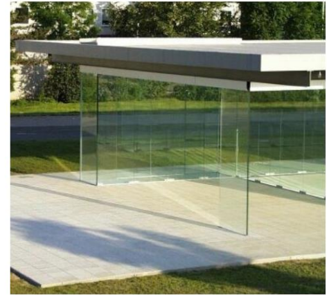
Figure 9: Use of glass as primary structural elements Centre of German Glazing Handcrafters in Rheinbach, Germany.
