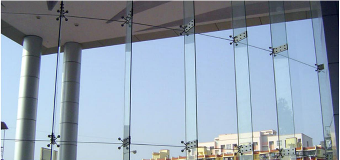
Figure 1: Structural Bolted and Clamped Assembly Applications
